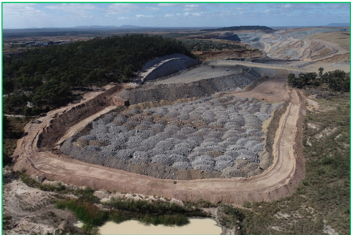
Figure 5: Drone view of recent backfilling in M Pit.
