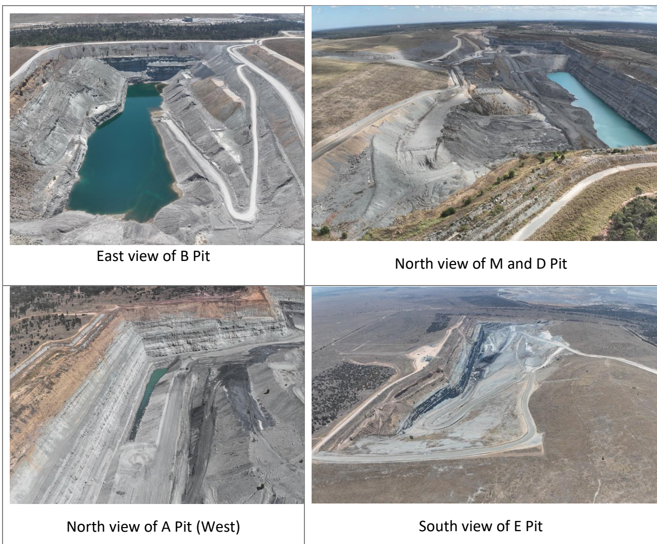
Figure 3.1 Aerial photographs of the existing open cut mining pits considered in the assessment
