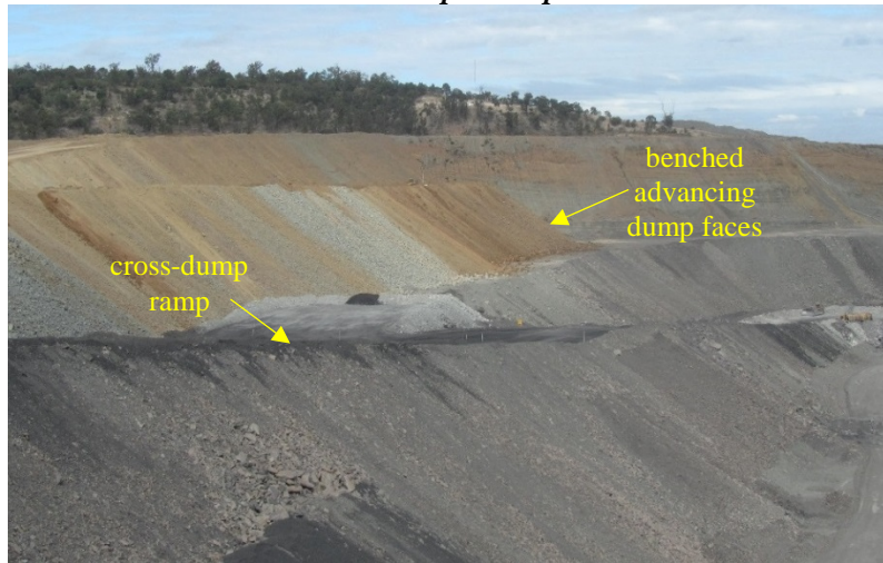
Photo taken 9/05/2017, looking SW
